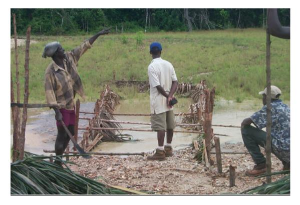
Photo 18 - Damming of Arakaka Creek by Confining Tailings Discharged Directly Between Two Rows of Plaited "Cocorite" Leaves Supported by Stakes.
