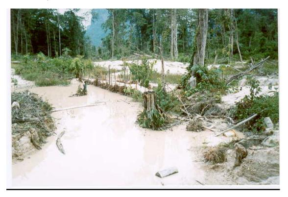
Photo 16 – Construction of Tailings Confinement Dam From Indigenous Material, as Part of a Closed Circuit System at Upper Takuba Creek.
