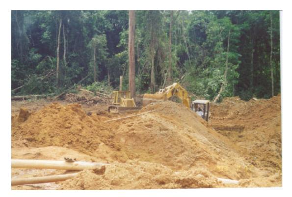
Photo 23 - A Small Cat. Dozer, at Five Star, Enabled Better and Safer Ground Preparation as well as some Land Reclamation.
