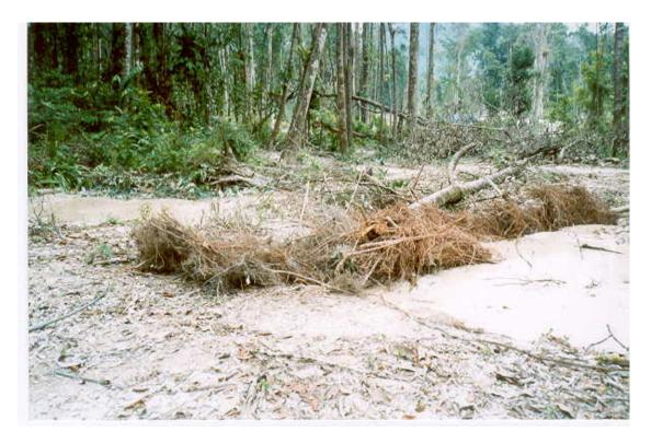
Photo 17 – A Filtration Dam Constructed From Fibrous Roots and supported by Tree Trunks, as Part of a Closed-Circuit Recycled Water System at Upper Takuba Creek.
