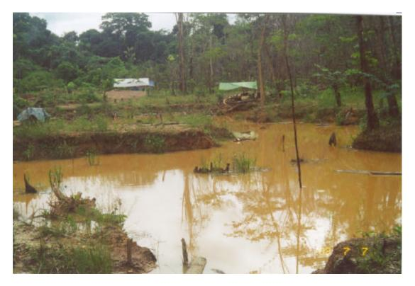
Photo 20 - Tailings Impoundment System Employed at 10 Miles, where Tailings is Routed Through Mined-Out Pit allowing Partially Settled Water to be Decanted to Nearby Stream.
