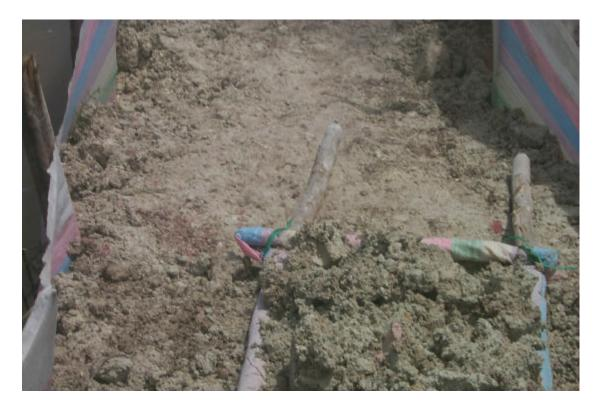
Photo 2 - GGMC's EXPERIMENTAL DAM - Core Fill Between Filter Linings
