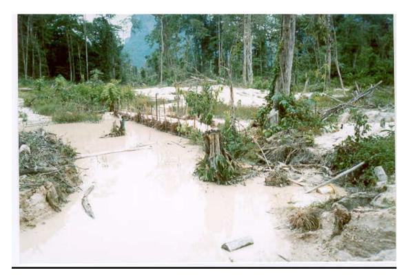
Photo 7 – Construction of Tailings Confinement Dam From Indigenous Material (as Part of a Closed-Circuit System) at Raimundo DaSilva's Operations at Upper Takuba Creek.
