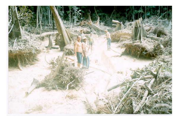
**Photo 3 -** Unique Land Dredging Operation (by Carlos DeAguiar at Barlow) where a Cluster of Tree stumps Left in Place After Jetting Operations.
