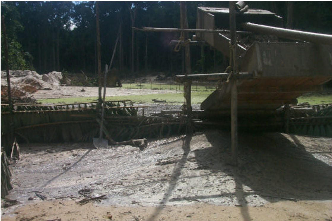
Photo 14 – Typical sluice box set, G. Costa’s operation at Baramalli.
