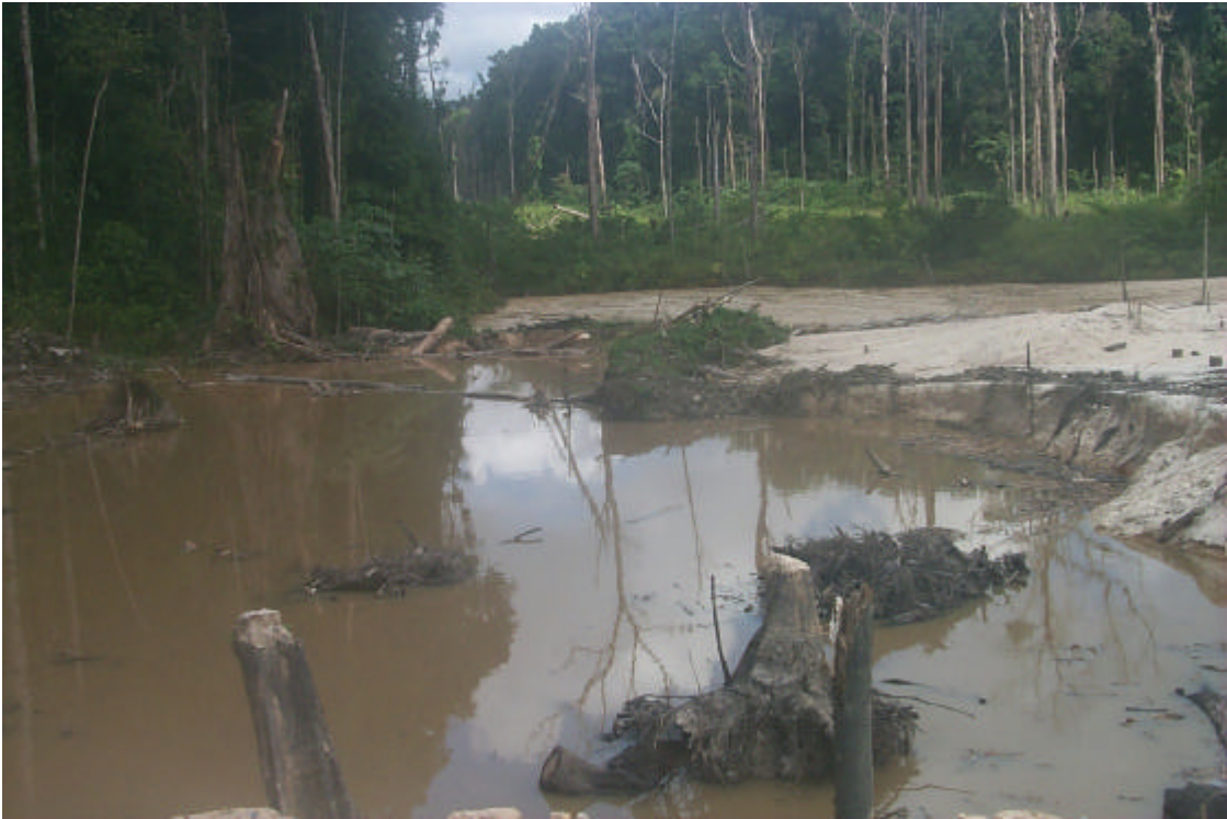
Photo 3 – Old mined-out pit being backfilled, N. Hopkinson’s operations at Quartz Stone.
