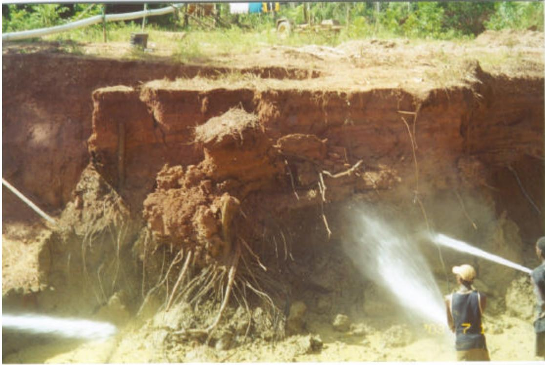
**Photo 3** - A Typical Land Dredging Operation (by Brian Phillips at Arakaka) where both Overburden and Pay Material are Removed by Jetting and Routed Through Sluice Box.
