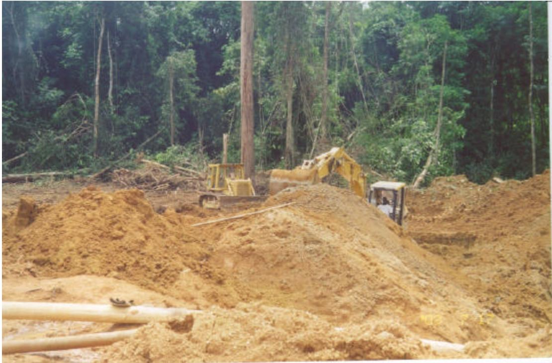
**Photo 7** - The Impact of Mechanization: The use of Small Cat. Bulldozer (C. Adams' Operation at Five Star) Enables Better and Safer Ground Preparation as well as some Land Reclamation.
