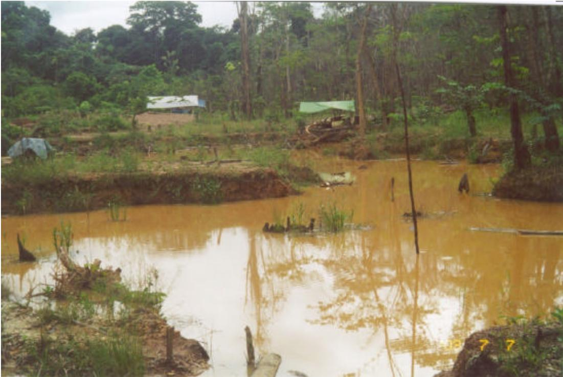
**Photo 1** - System of Tailings Impoundment Employed by the Rodrigues at 10 Miles where Tailings Discharge is Routed Through Mined-Out Pit then Partially Settled Water Decanted to Nearby Stream.
