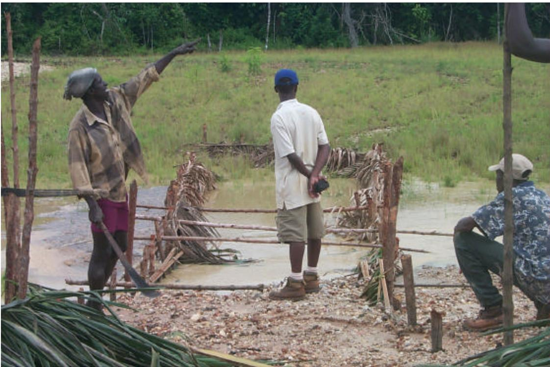
**Photo 2** - Damming of Arakaka Creek (by Older Method of Confining Tailings Discharged From Sluice Box Directly Between Two Rows of Supported and Plaited "Cocorite" Leaves) In-order to Reroute Creek Flow to Allow Mining of Current Creek Bed.
