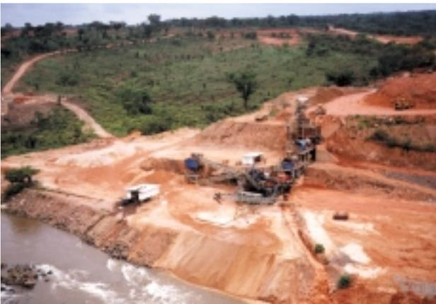
*A complete diamond recovery plant in Angola incorporating a 50 t/h DMS module.*
