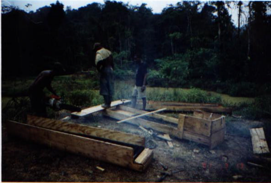
Photo 19 – Construction of Peter Thompson's New Sluicebox
