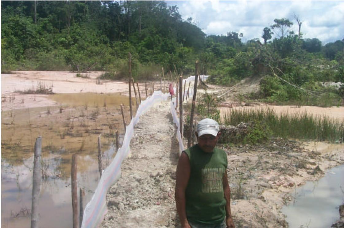
**Photo 19** - GGMC's Experimental Dam – Local Filter Linings Pinned by Wooden Stakes
