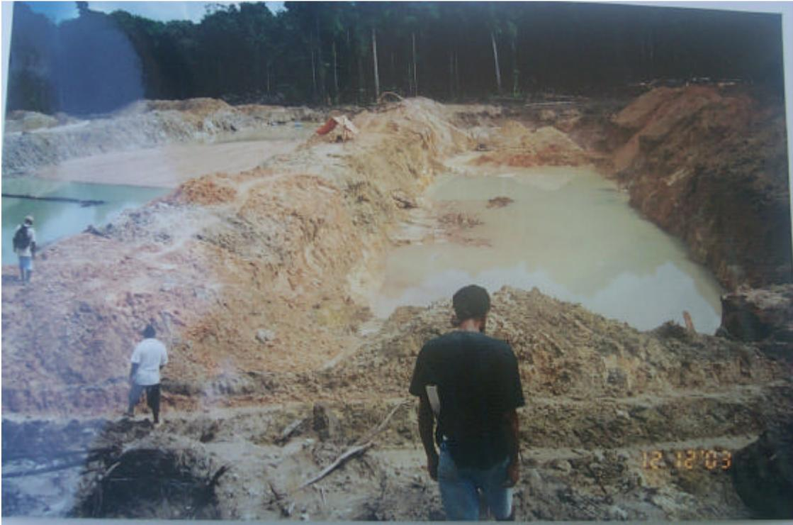
**Photo 13** – Good pit configuration with, well-defined pit faces at Middle Aremu. Note, vertical pit faces (25 to 30ft.) deep with overburden overcastted close to the edge of the mining face.
