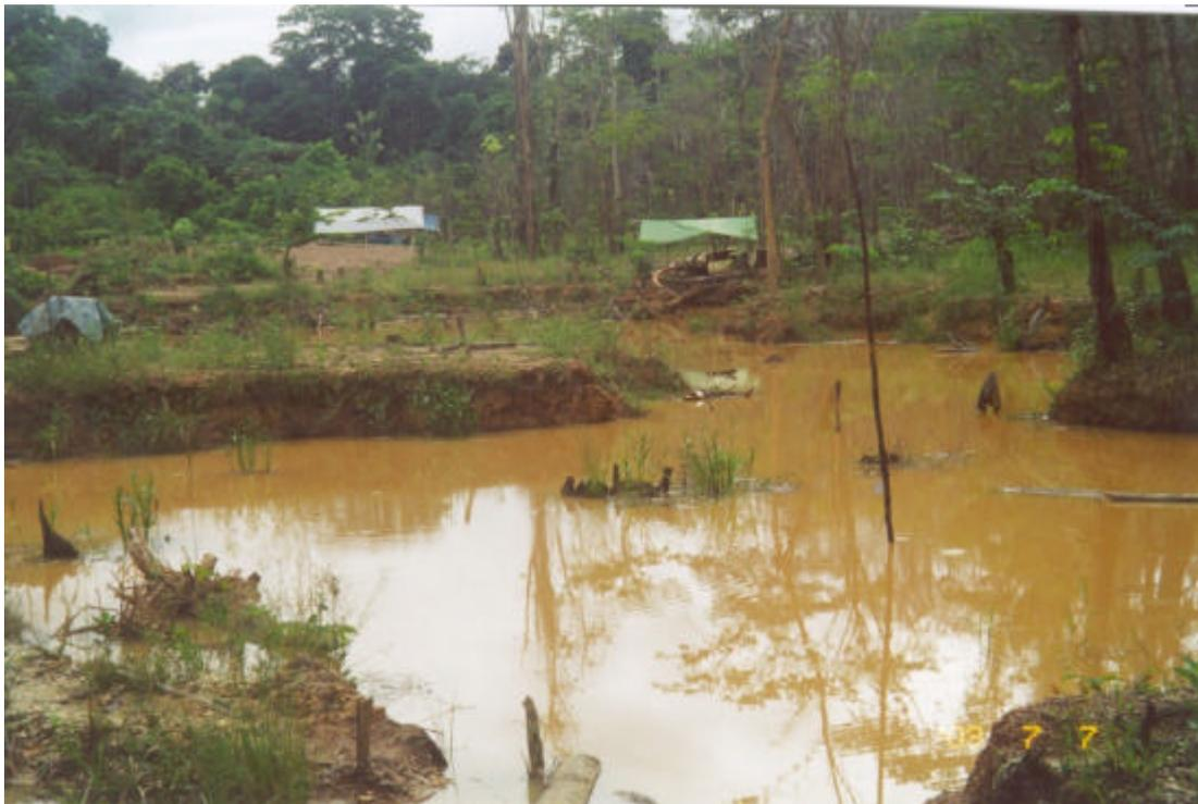
**Photo 20** - Tailings Impoundment System Employed at 10 Miles, where Tailings is Routed Through Mined-Out Pit allowing Partially Settled Water to be Decanted to Nearby Stream.
