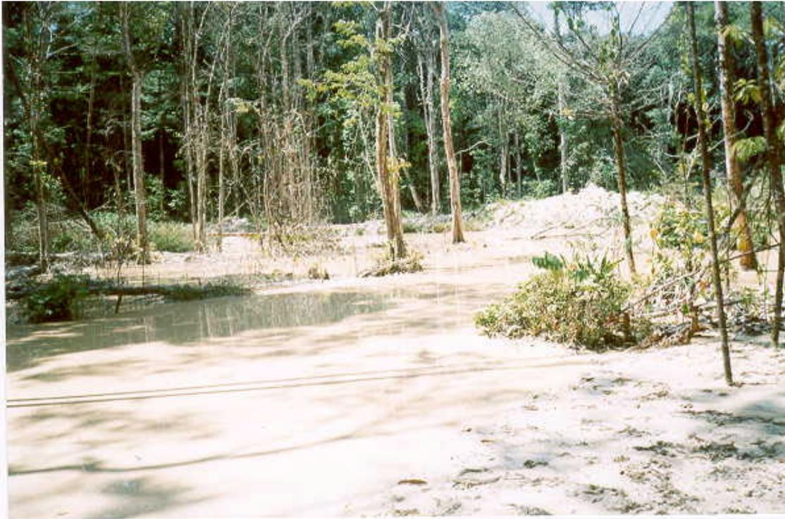
**Photo 15** – Tailings Confinement Dam as Part of The Closed Circuit Recycled Water System at Barlow.
