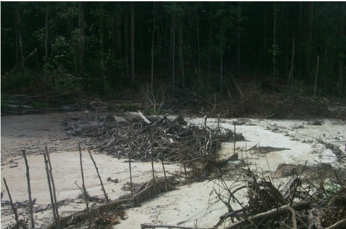
**Photo 14** – Crude system of indigenous material used to confine tailings solids at Baramalli.
