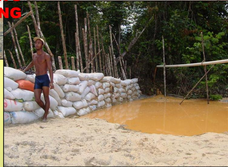
Using local materials plus imported sand bags a large breach to the river is dammed. The idea is that **coarse tailings** will accumulate further back from the dam wall with the aid of **silt fences**. Suspended material in the water (**fine tailings**) held back by the dam will then have time to settle before discharging to river.
