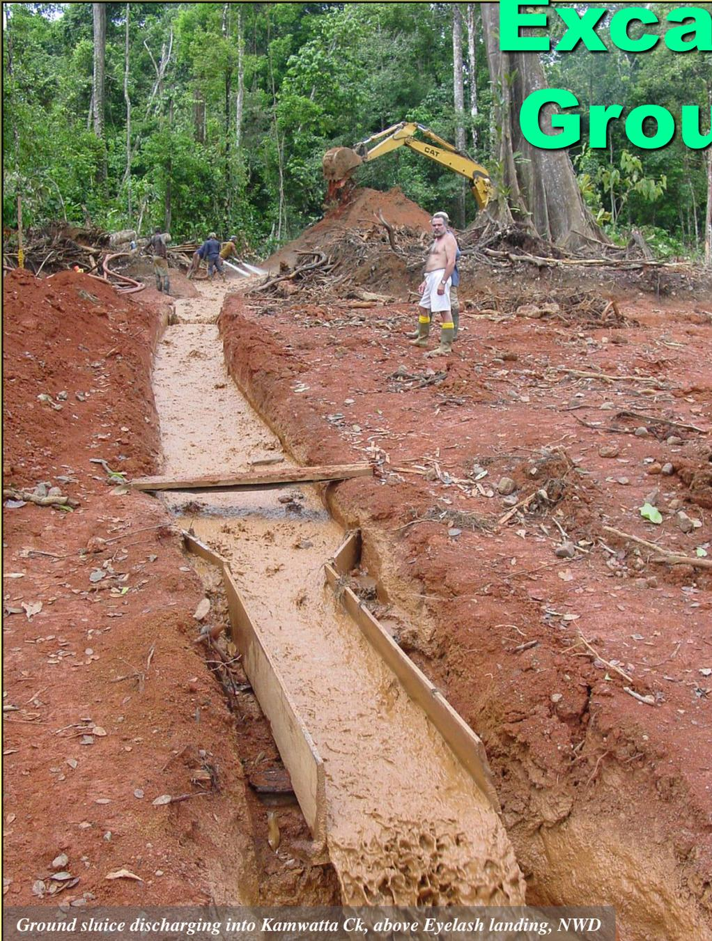
*Ground sluice discharging into Kamwatta Ck, above Eyelash landing, NWD*
