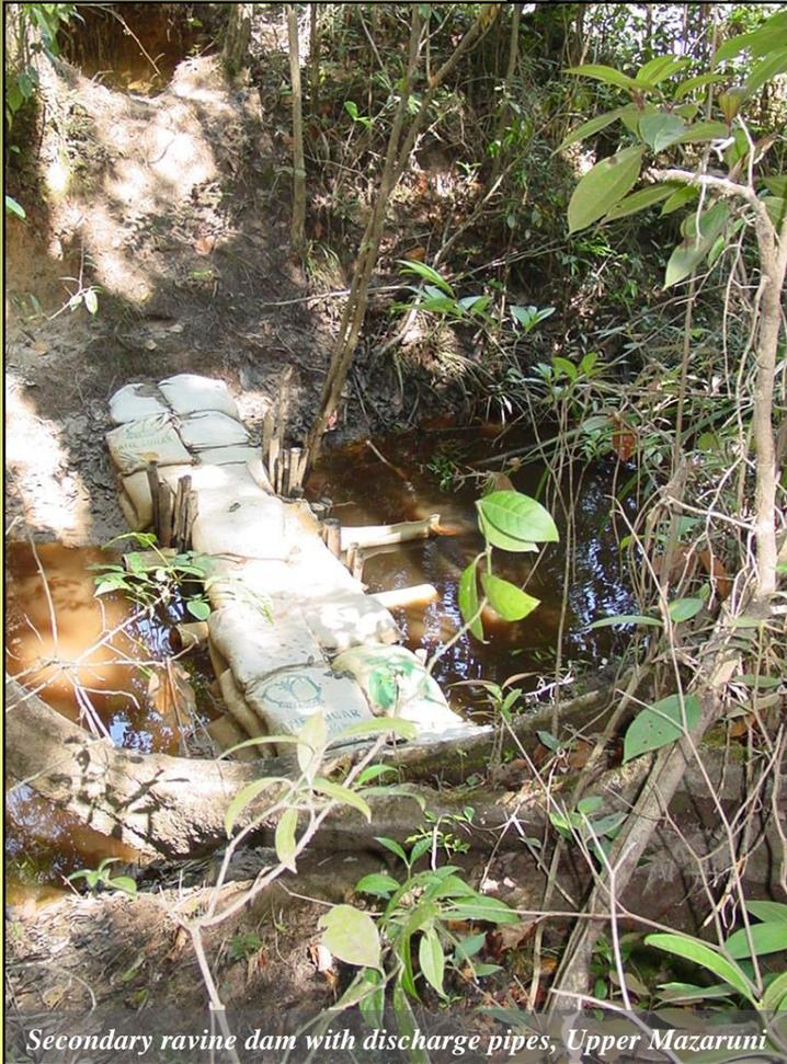
Secondary ravine dam with discharge pipes, Upper Mazaruni
