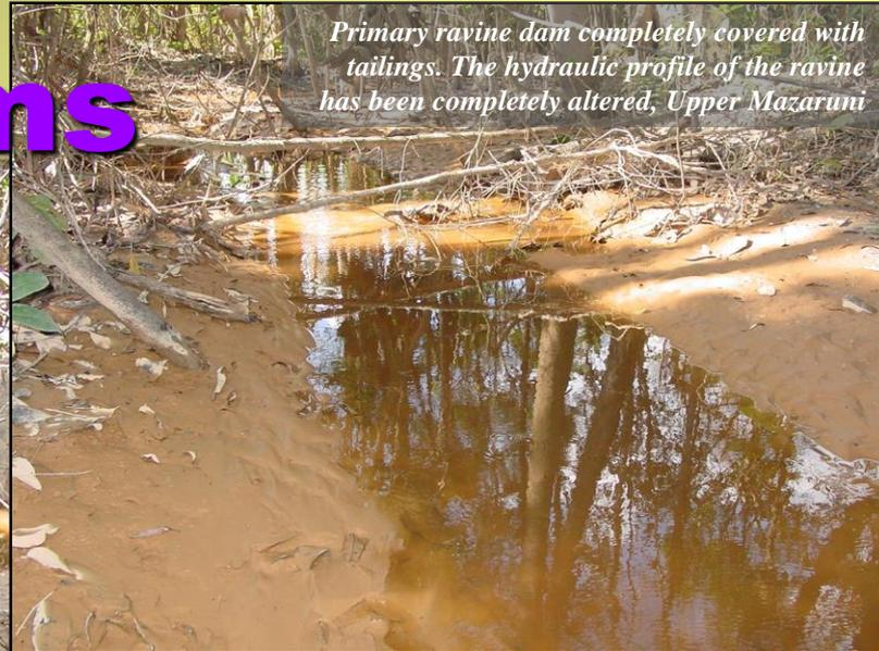
*Primary ravine dam completely covered with tailings. The hydraulic profile of the ravine has been completely altered, Upper Mazaruni*
